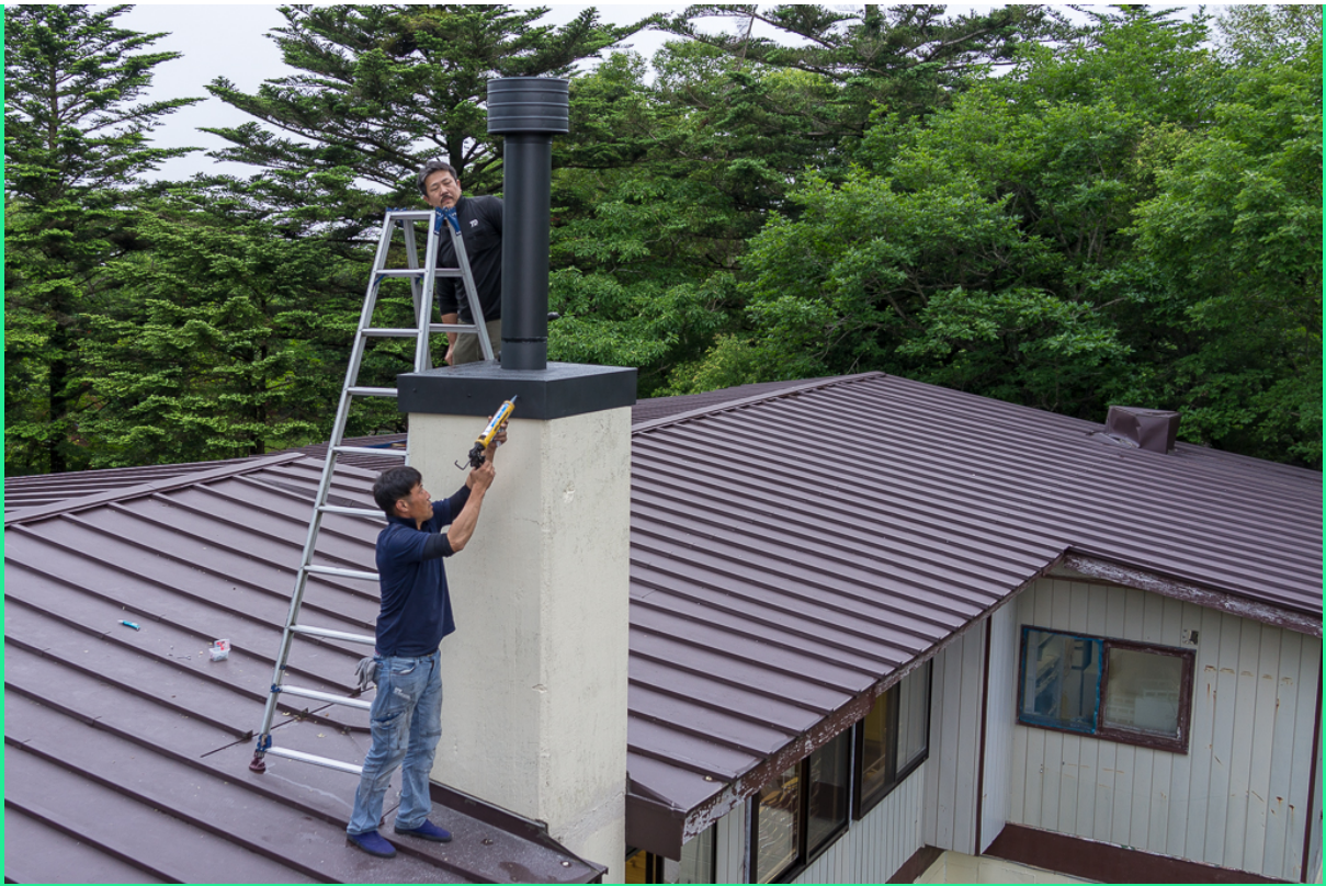
Finishing the new chimney that passes thru the old fireplace chimney.
